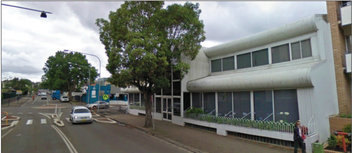
Photograph 10: View of commercial building to the immediate north of the subject site along Villiers Street, looking north.
