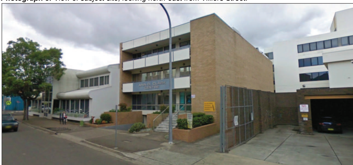
Photograph 4: View of north-western corner of the subject site from Villiers Street, looking east.
